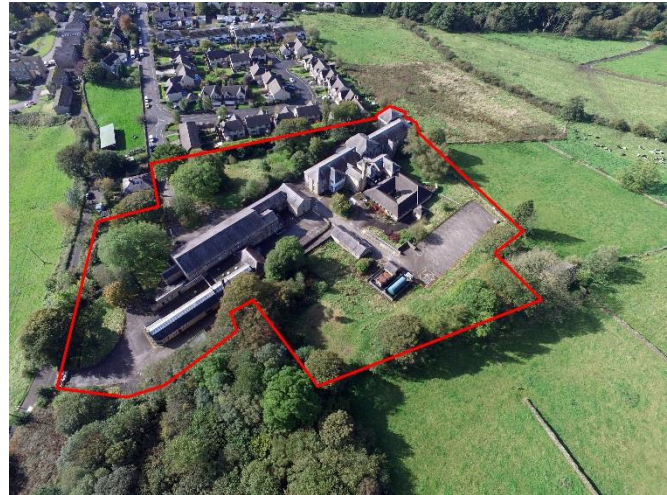
Aerial of existing buildings looking south
