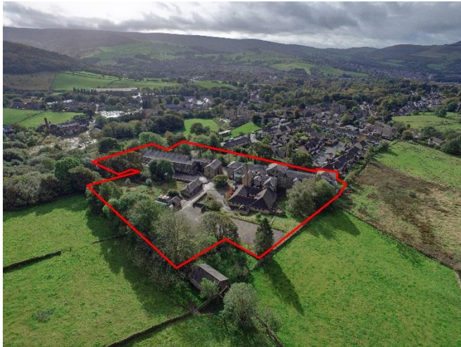
Aerial of Planning Application Plan Area looking east
